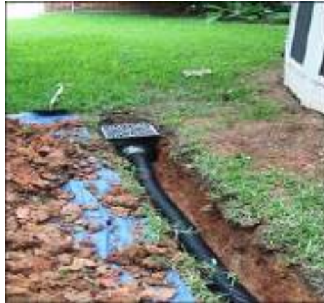
Fig 2. Buried Pipe Drain
