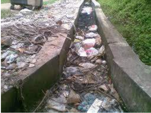
Fig 4 (a) Blocked Drains
