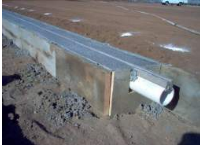
Fig 3. A Slot Drain System (Source: sportsedge.com)
