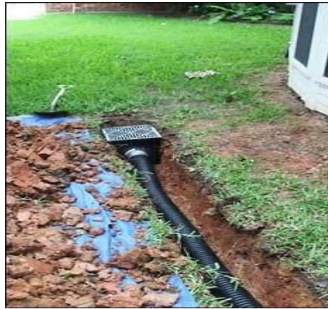
Fig 2. Buried Pipe Drain
