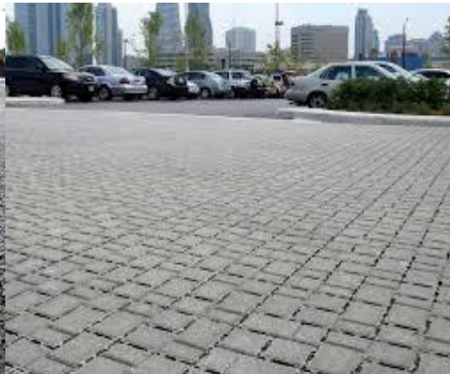
Fig 6 Interlocking concrete (Source: 3driverswetweather.org)
